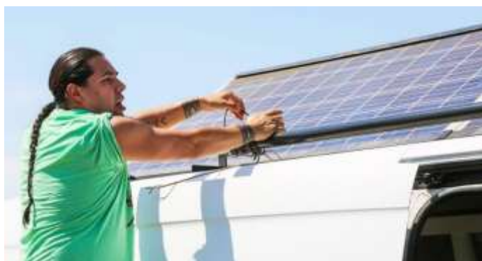
Installing solar panels
